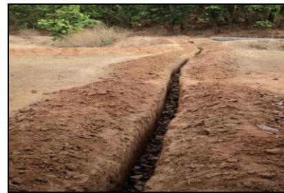
Channel for inlet pipe
