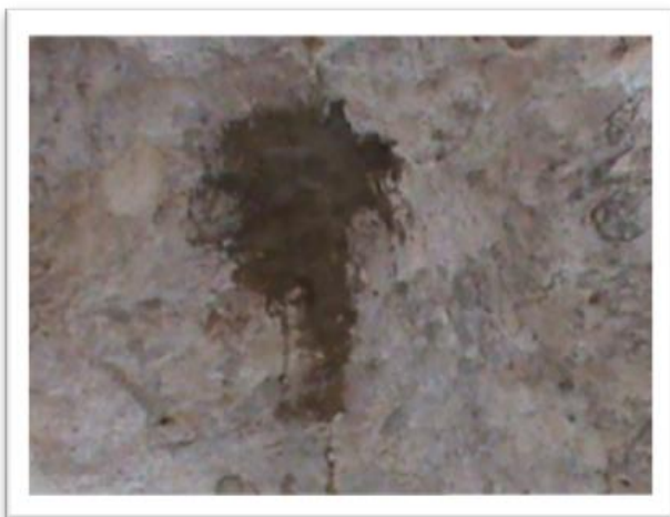
3. Covering the hole by moistened clay
