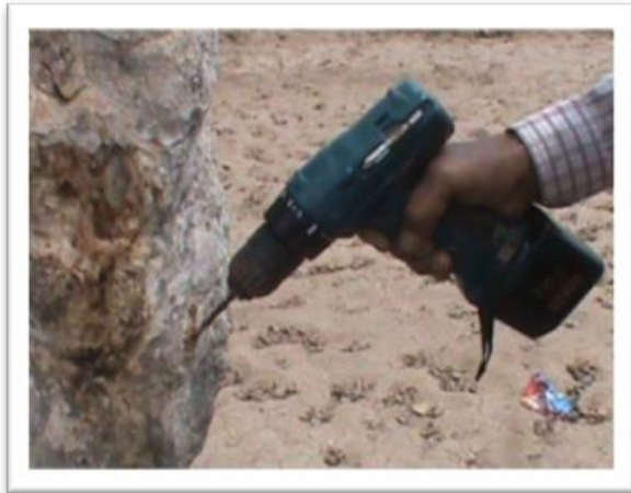
1. Making hole with battery operated drill
