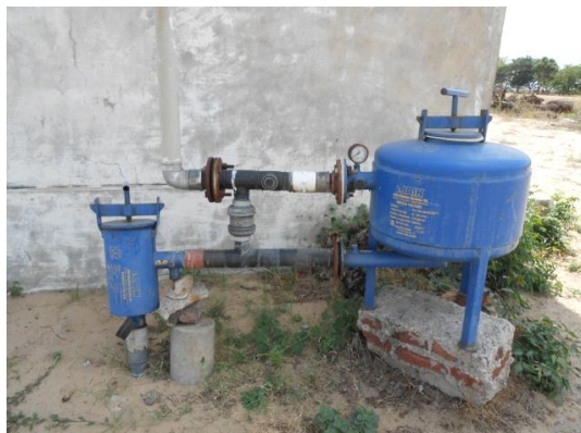
Plate 1: Water distribution system with sand filter, screen filter and other accessories
